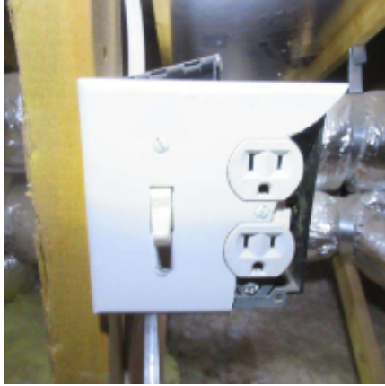
Image 3.4.1 Broken Outlet Cover
