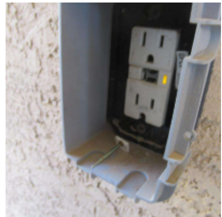
Image 3.3.3 Broken GFCI Test Button
