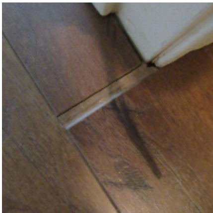
Image 6.1.1 Hardwood Flooring Gap - Master Bdrm Entry
