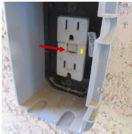
Image 3.3.2 Broken GFCI Test Button
