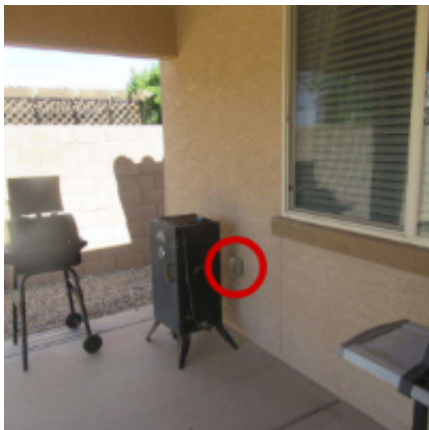
Image 3.3.1 Broken GFCI Location
