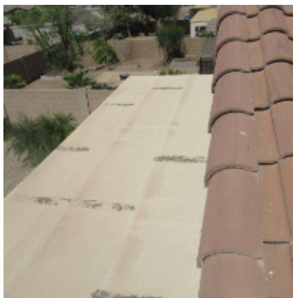
Image 2.2.2 Peeling coating from joints on patio roof
